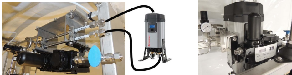
Figure 30 Instrument air dryer. External mount (left) and Internal mount (right).
